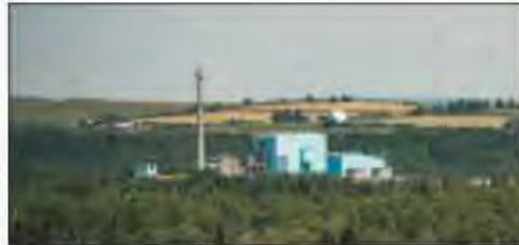
ReEnergy facility in Fort Fairfield, ME
