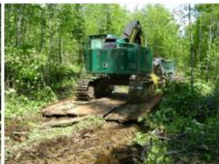
A temporary bridge.
