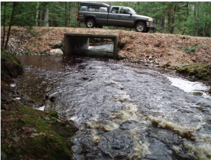
Photo 3.1 Box culvert installed in 2006 in compartment C
